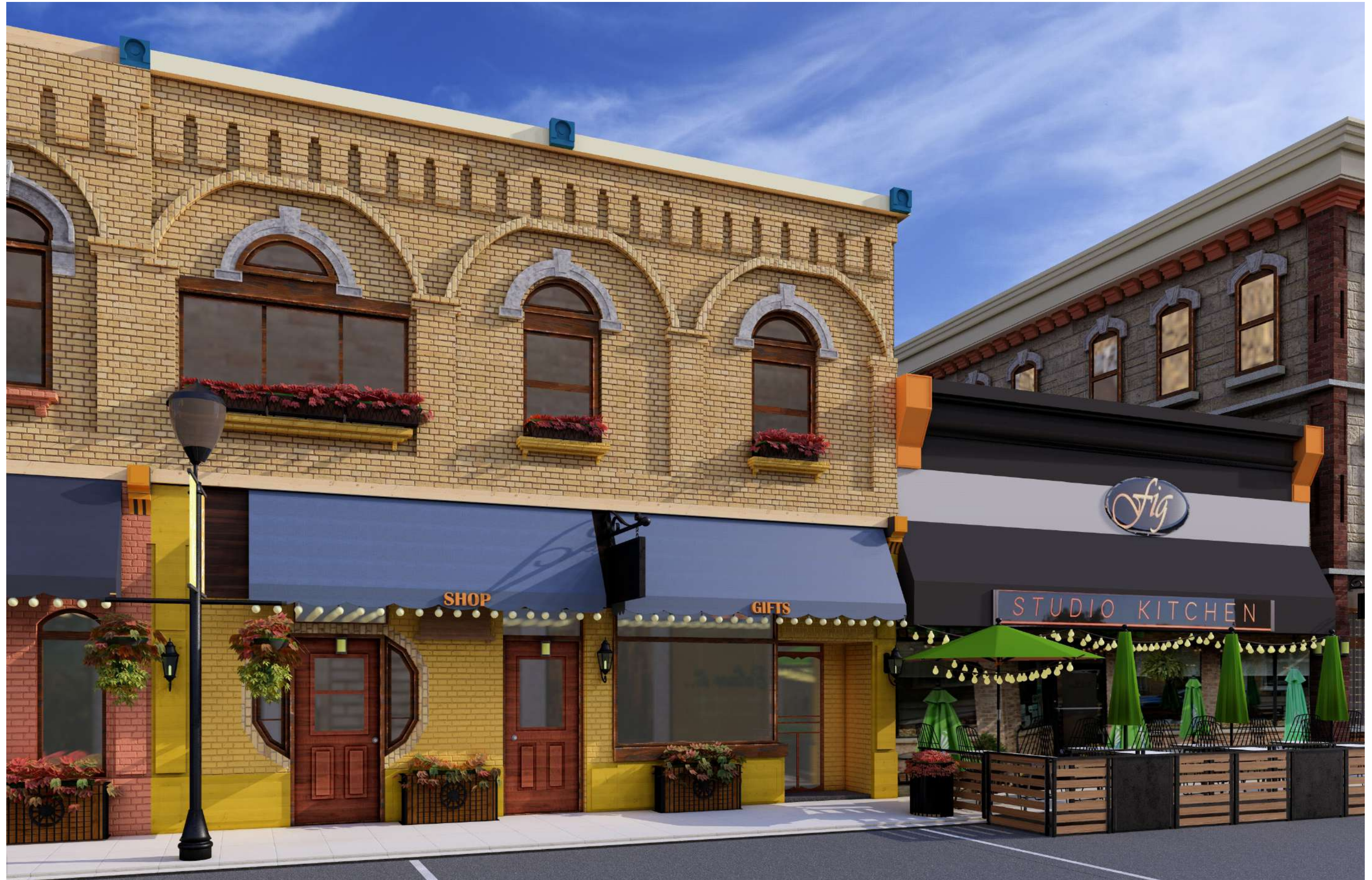
Façade enhancements at 83 Huron Street
