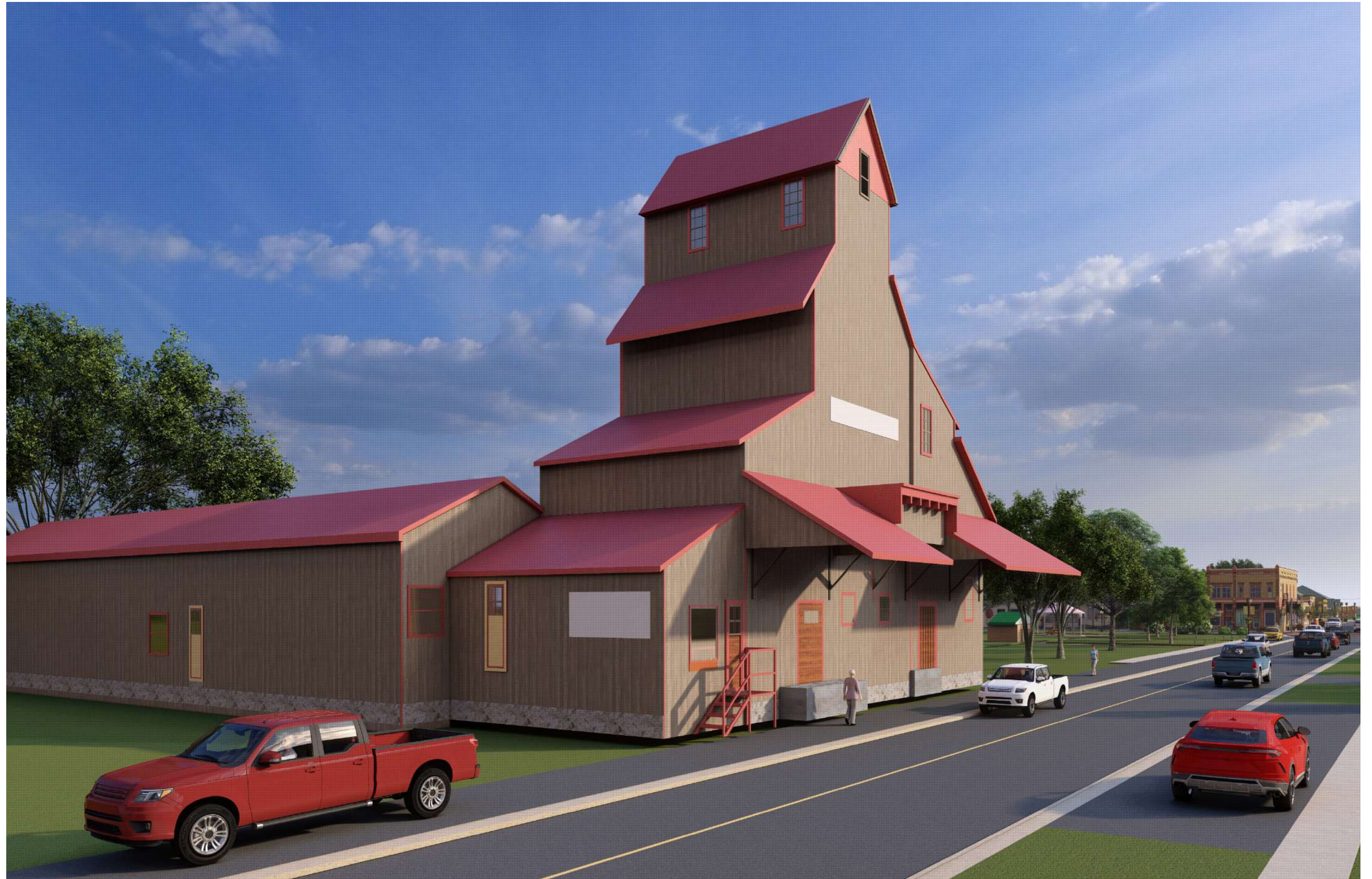
Restored Henshall Co-Op Building
