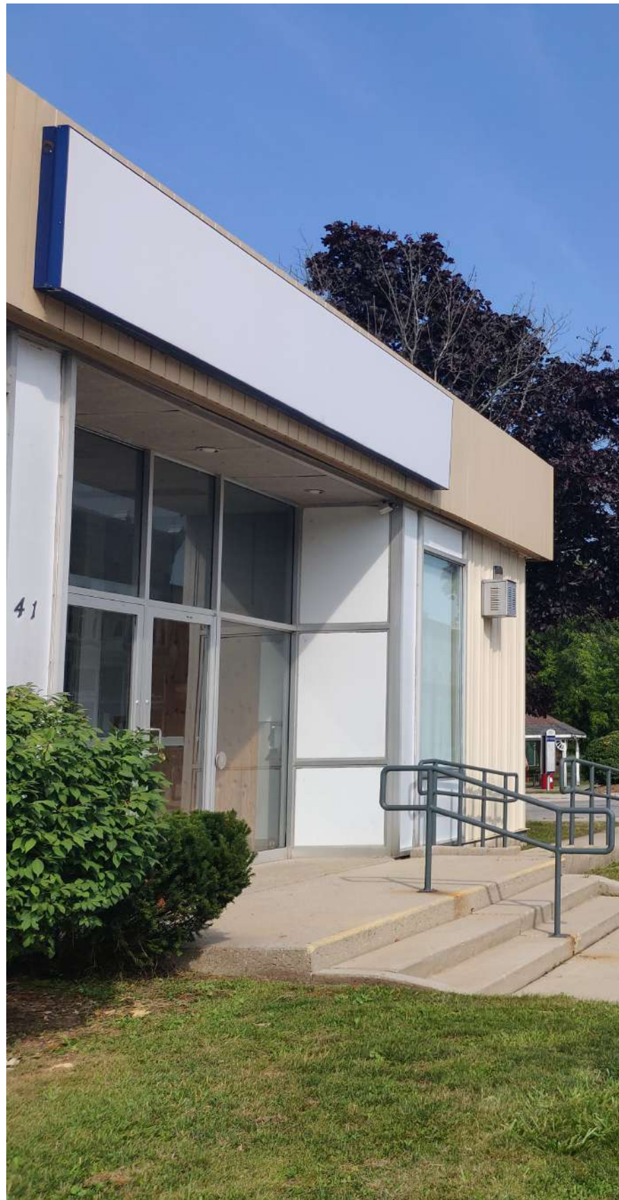
The Old Bank on Queen Street
