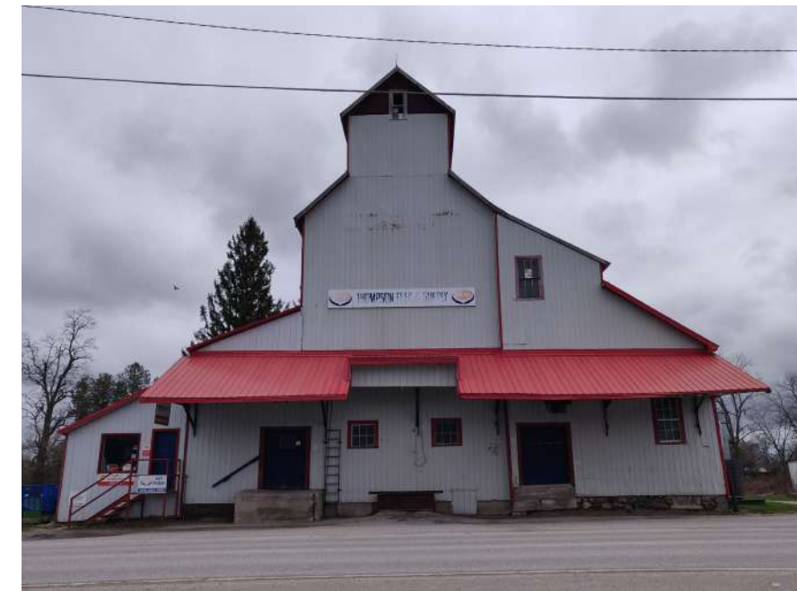
Reimagine vacant buildings - Henshall Co-op
